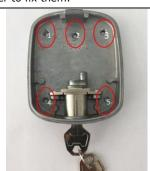
4. Punch 5 holes of ø6mm in the marked place and then install expansion screw
